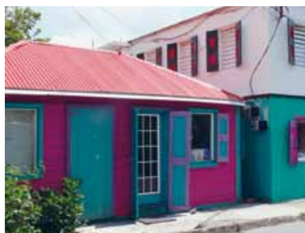
Casa a Road Town
